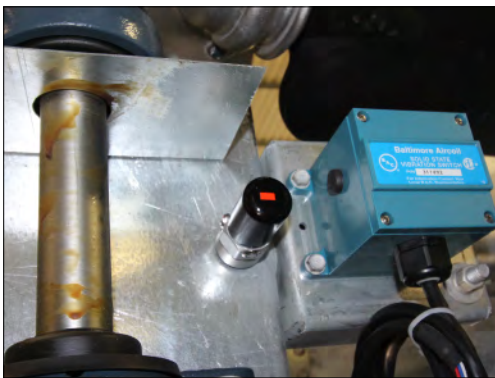
Figure 11a. Preferred Accelerometer Location
