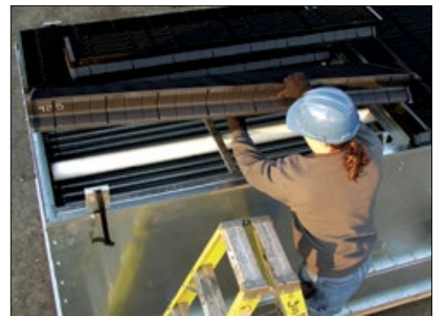
Inspecting Drift Eliminator
