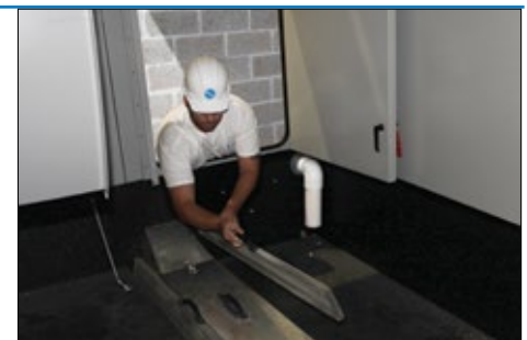
Inspecting a Cold Water Basin Strainer
