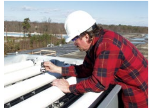
Inspecting Spray Nozzles
