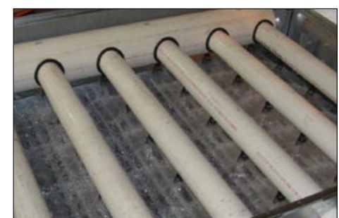
Pressurized Spray Water Distribution
