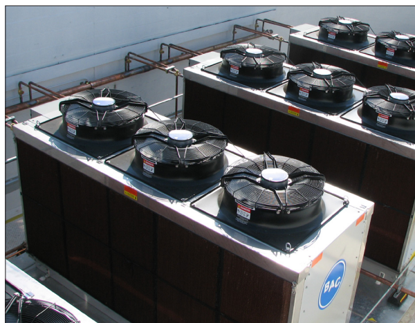
TrilliumSeries™ Condensers Purchased in California Due to their Reduction in Energy Use Compared to Air-Cooled Condensers
