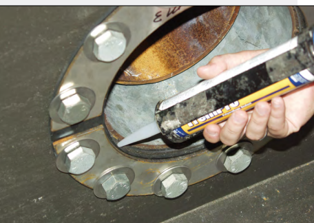
Figure 13. Caulk Exposed Galvanized Steel
