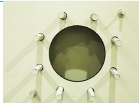
Figure 4. An ASME Class 150 Flat Face Flange Pattern with Mounting Bolts is Shown on this Hot Water Basin Panel
