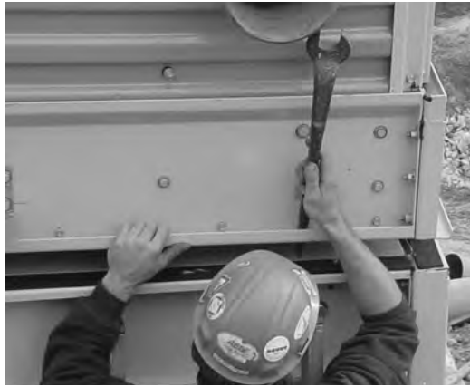
Figure 5. Drift Pin Alignment
