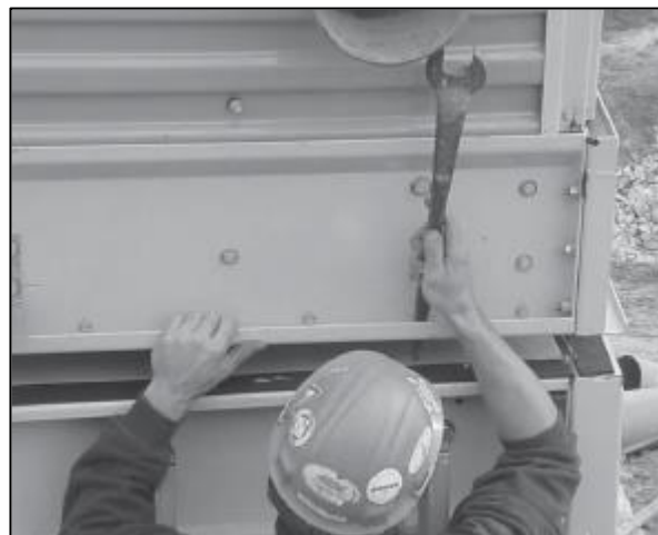
Figure 4. Section Alignment Using Drift Pins
