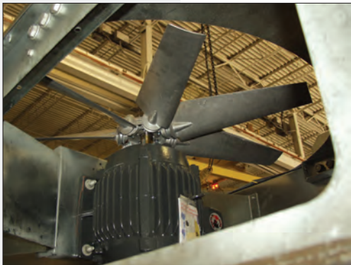
Figure 2a. Direct Drive Motor
