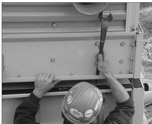
Figure 4. Drift Pin Alignment
