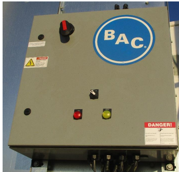
Figure 22. EC Fan Control Enclosure for Models VRC-xxxxA-xxxxN-xB
