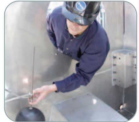
Figure 3 - Water Make-up Valve Assembly
