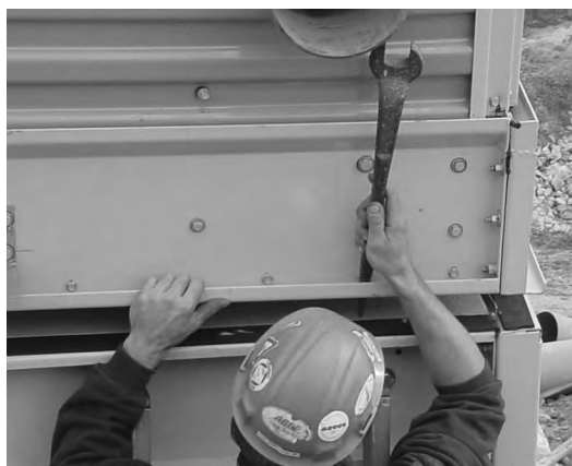
Figure 4. Drift Pin Alignment
