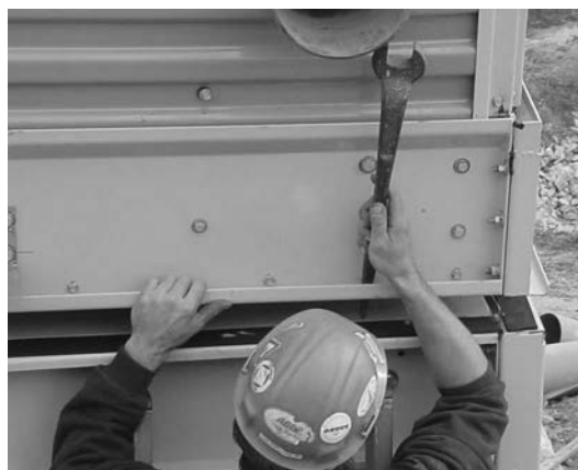
Figure 4. Drift Pin Alignment
