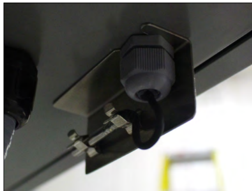
Figure 29. Ambient Temperature Sensor
