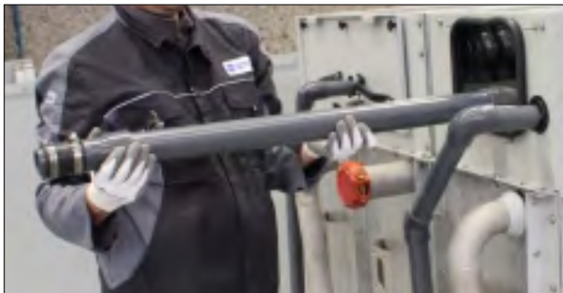
Figure 24. Spray Branch Removal
