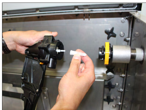
Figure 19. Mechanical Make-up Valve Assembly Filter Cleaning
