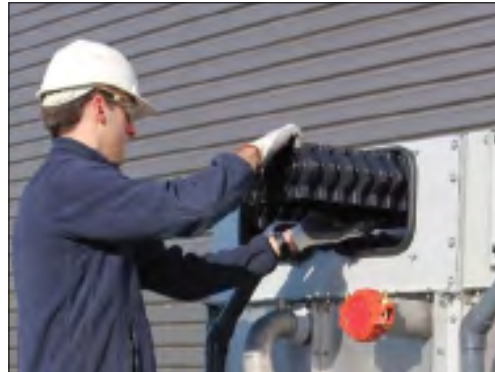
Figure 25. Drift Eliminator Removal
