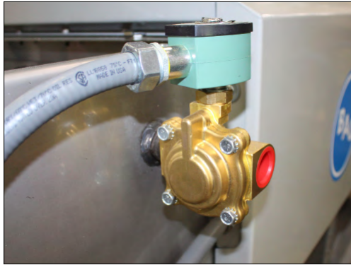
Figure 27. Solenoid Make-up Valve
