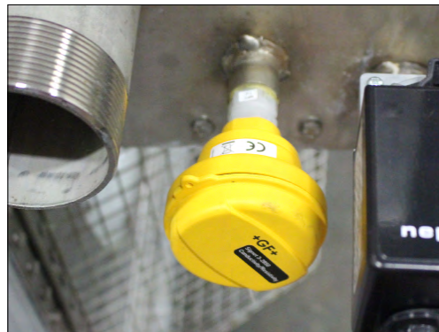
Figure 30. Conductivity Sensor
