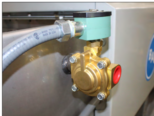
Figure 40. Drain Solenoid Valve
