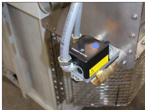
Figure 21. Drain Valve
