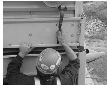
Figure 6. Drift Pin Alignment
