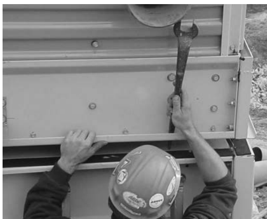
Figure 4. Drift Pin Alignment
