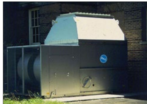
Series V Centrifugal Fan Single Side Air Intake Unit with Full Sound Attenuation
