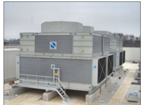
An Evaporative Condenser with Full Sound Attenuation
