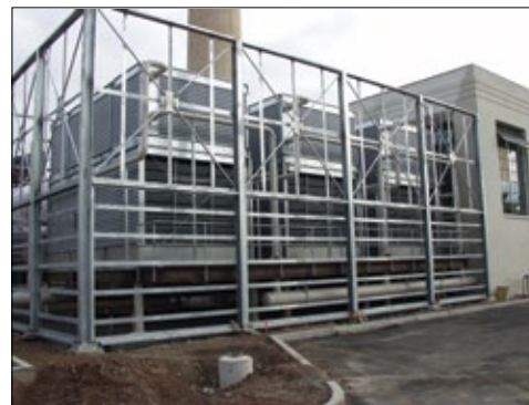
Barrier Walls Being Erected Around FXV Dual Air Intake Units
