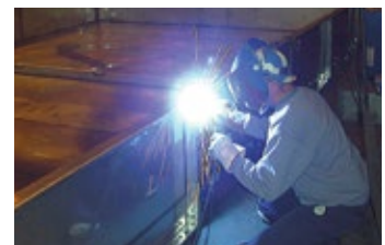
Basin Seams are Welded
