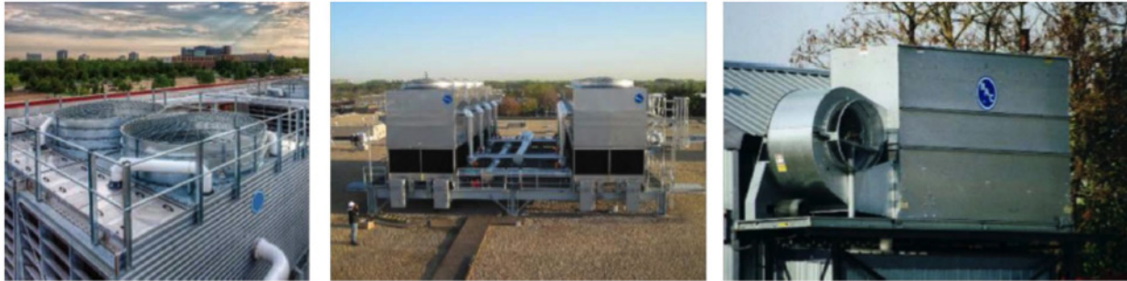
Figure 11 Open Circuit Cooling Towers Available in a Wide Variety of Sizes and Configurations
