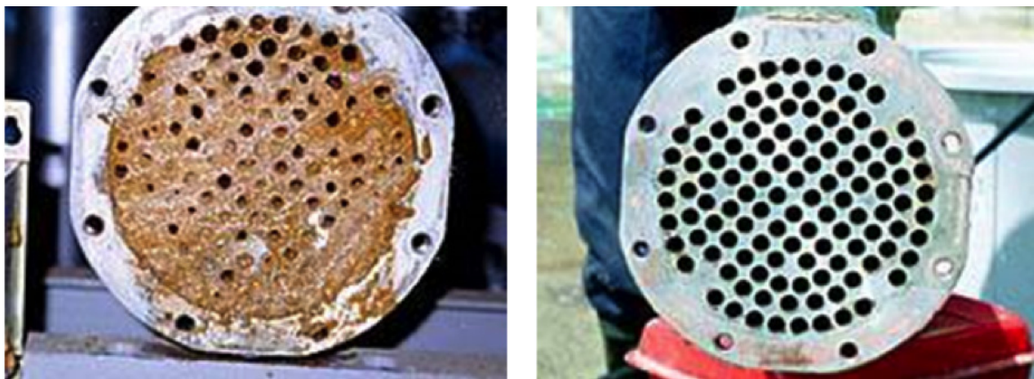
Figure 5 Shell & Tube Heat Exchanger Before and After Cleaning
