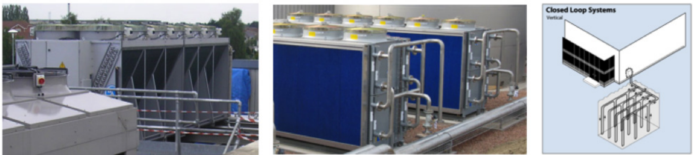
Figure 7 Some Options to Close the Loop - Dry Cooler, Adiabatic Fluid Cooler, and Ground Source Heat Exchanger, Respectively
