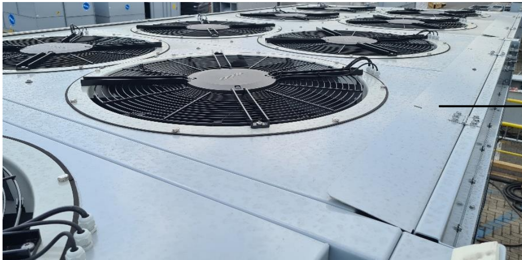
Figure 11. Upper water distribution channel inspection cover
