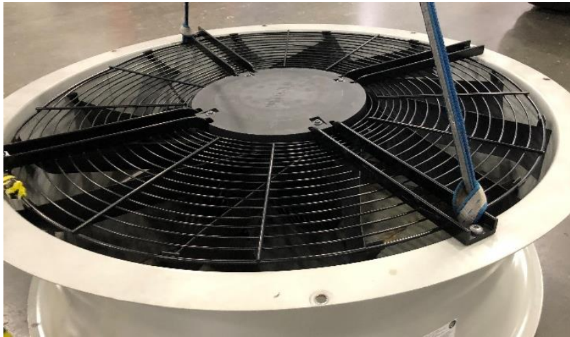
Figure 23. Fan and Motor Assembly Lift
