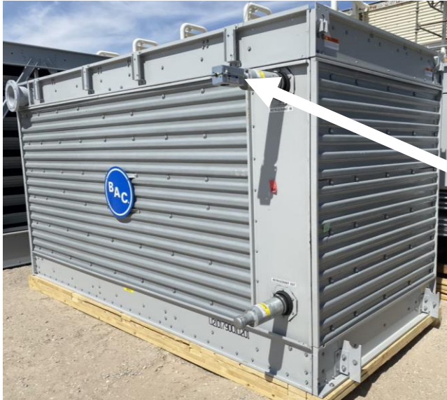
Figure 27. Coil Connections Capped and Charged
