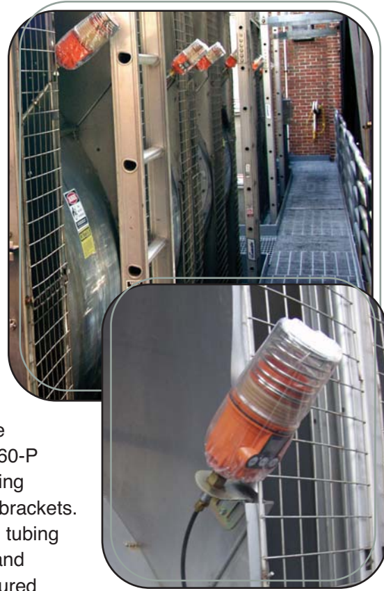
Typical Bearing Greaser Installation
