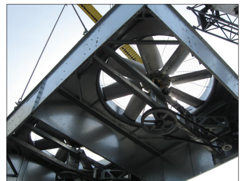
BALTIDRIVE® Power Train Fan System Used for VFD Applications
