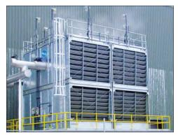
External Ladder, Safety Cage, and Handrail
