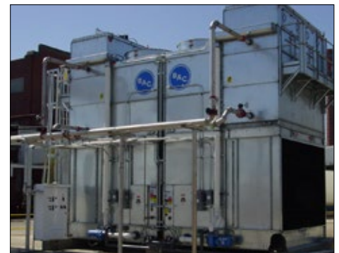
Fluid Cooler / Closed Circuit Cooling Tower
