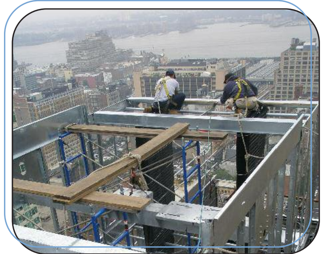
Installation of Knockdown Cooling Towers
