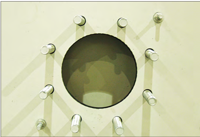
Figure 4. An ASME Class 150 Flat Face Flange Pattern With Mounting Bolts is shown on this Hot Water Basin Panel
